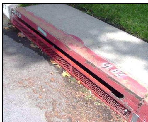
Figure 2. CB curb opening screen, fixed
